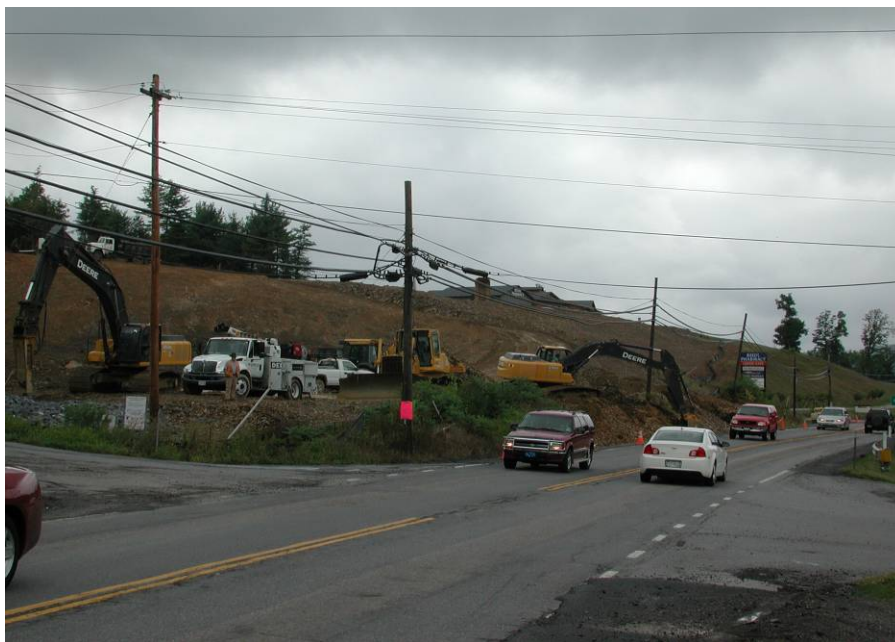
Figure 18: Construction in the watershed
