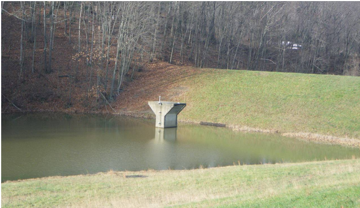
Figure 13: Flood control structure
