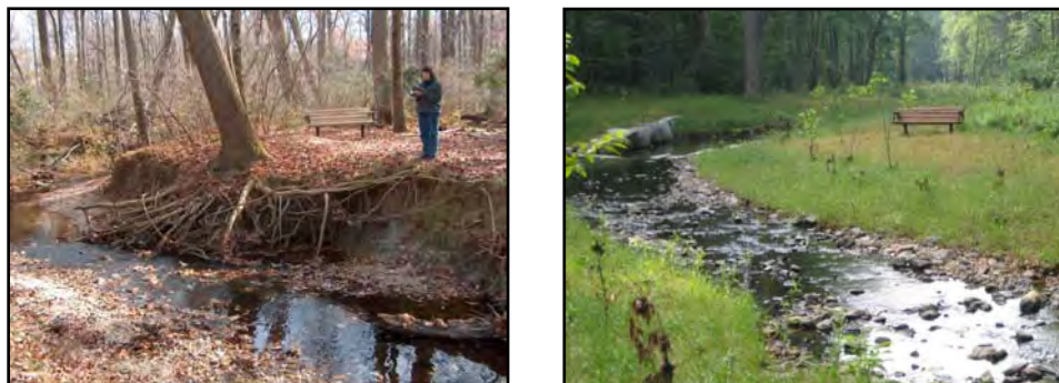
Figure 21 A/B - Snakeden Branch, Reston, VA. Invert raised to reconnect to the floodplain.
