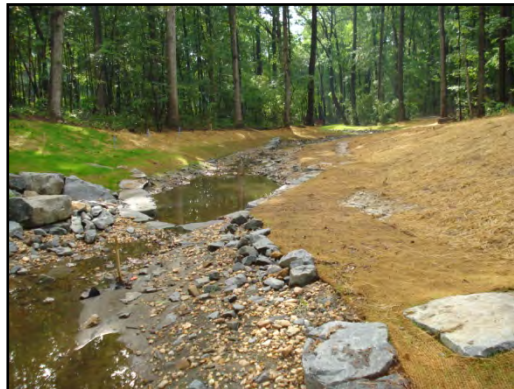
Figure 25 - Snakeden Branch, Reston VA. Newly constructed bankfull bench at lower elevation.
